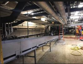
Justin Mayfield and Ben Houchin working to install stainless steel piping for 36 motors and disconnects that are in the lower rendering area of Tyson Fresh Meats. There are many challenges in this area including low ceilings, open conveyors,
