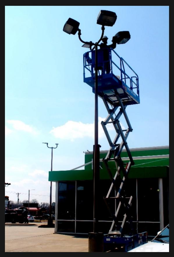
Jon Spivey from the Decker Electric service department is currently working on the Enterprise Rental Car Sales Lot in Wichita, KS. Scope of work includes replacing (66) 1000 watt metal halide fixtures with 300 watt LED flood fixtures. The project is scheduled to be completed by April 10th.
