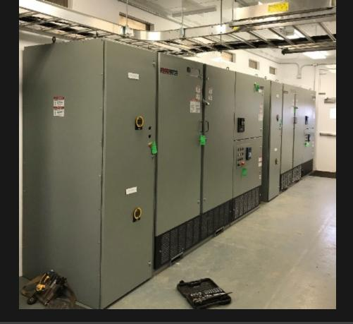
James Eck, John Ramey, Darren Wilcox and Mason Smith, with assistance from Minnesota Limited, installed two 1250HP VFD's inside an elevated electric building on the Enbridge Booster Pump project in Cushing, OK. Each weighed just over 12,000 pounds,
