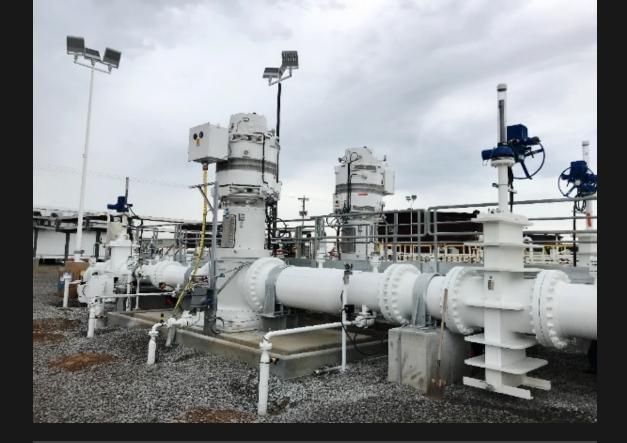
Project included installation and new power service to two new 4160-volt VFDs. The motors pictured above are being serviced by VFDs. In addition, we provided and installed a full UPS system, heat trace system, site lighting, cable tray, and instrumentation wiring. The project also required the construction of a relay cabinet, fiber back bone, and LV power. Thanks to foreman, James Ek, and his crew and general contractor, Minnesota Limited.
