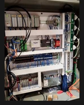
Decker engineered and supplied a turn-key replacement control system for an existing ride at Hershey Park in Hershey, Pennsylvania. This included replacing the existing motor/generator DC drives with AC VFD systems.
