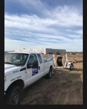
Dondlinger and Decker Electric are currently ramping up manpower as the Camping World and Gander Outdoor Buildings become "weathered in". Current construction involves temp power for roof-top units for temporary heat, service and mechanical wire pull, branch conduit for power and lighting and general purpose power for retail space and office areas. This fast-paced project is scheduled for completion mid-to-late May 2019.
