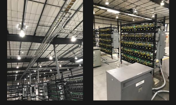
John Perkins, Jonathan Holdaway, Dave Wiley and others have been building a server for Aqua 305 in Wichita. Installing new panel feeders, branch circuits and wiring panels for the server racks to ensure the customer is up and running. Coordination between the City of Wichita, Westar and vendors has been essential to the success of the project.
