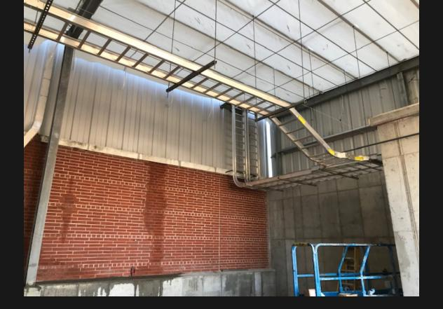
Foreman, Andi Krejci, Journeyman, Trent Potter and apprentices, Jake Baughman and Andrew Klump are staying busy at the Tyson facility in Lexington, NE. They are installing a carcass wash which rinses the sides of beef prior to curing. They are also installing new switchgear, cable tray, controls and lighting to prepare for new, more efficient gear. The job is scheduled for completion at the end of May.
