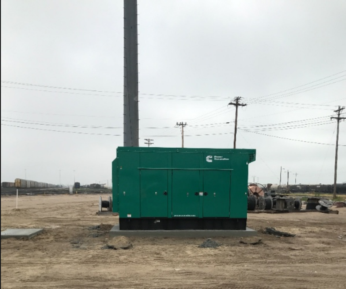
Bryan Wallace and Wayne Cooper successfully installed a 250kw Generator in North Platte, NE.
