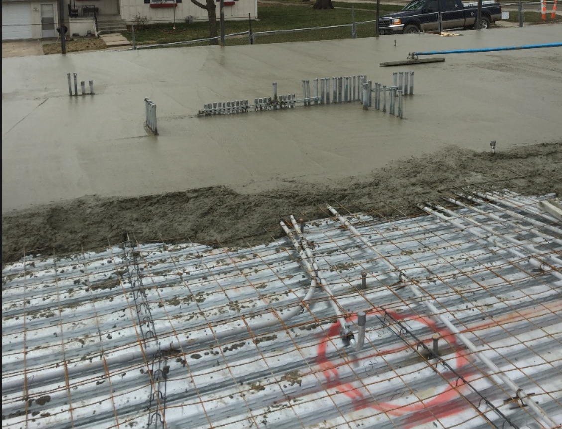
Slab rough-in on the 1st floor deck of the new Miami County Detention Center. Foreman: Brian Geist
